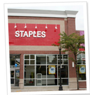
Our LEED Gold-certified store in Roslindale, MA, uses 35% less energy than the average Staples® store.
